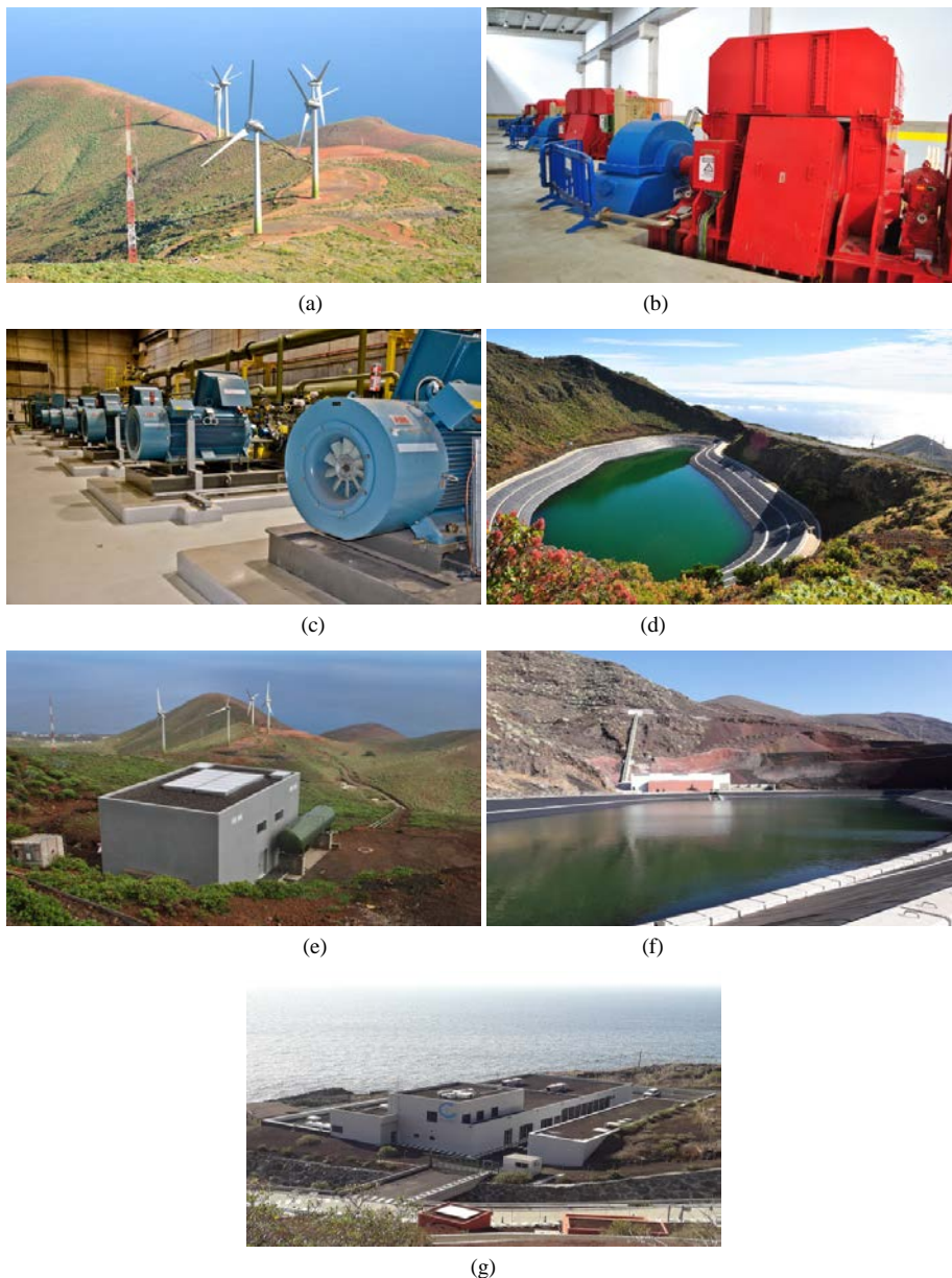
Figure 2. Gorona del Viento Wind-Hydro power plant: (a) Wind farm; (b) Hydro turbine station; (c) Pump station; (d) Upper reservoir; (e) Valve room of upper reservoir; (f) Lower reservoir; (g) Control, substation and pump station building.
