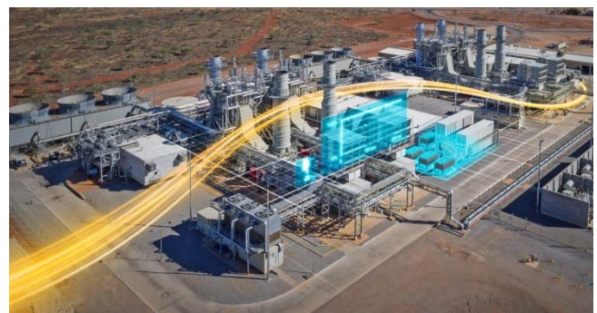
Figure 1: BESS collocated to a conventional gas turbine plant
