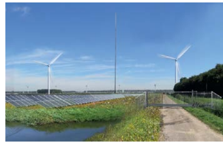
Fig. 5. The Haringvliet ; Vattenfall's first HPP combining wind, solar and battery storage since early development (Source: Vattenfall [14])
