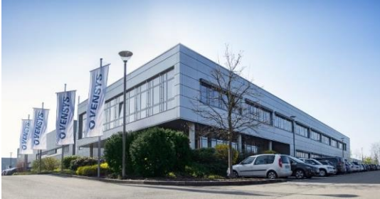
VENSYS Energy AG Headquarter - Neunkirchen (GER)
