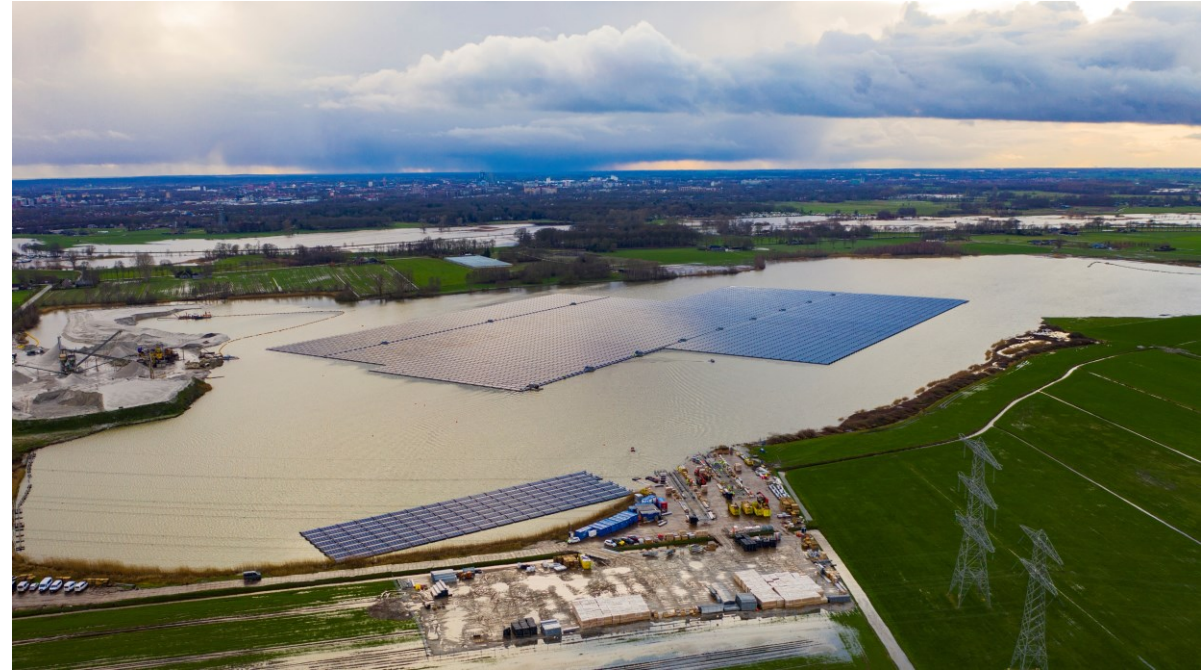
27 MWp in Netherland: Biggest floating PV plant outside of China, realized in only 7 weeks
