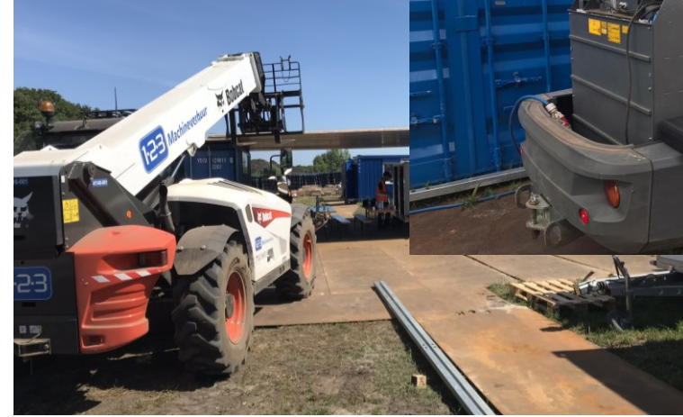
more electric machines on site
