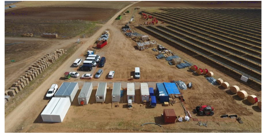
site with office and working containers
