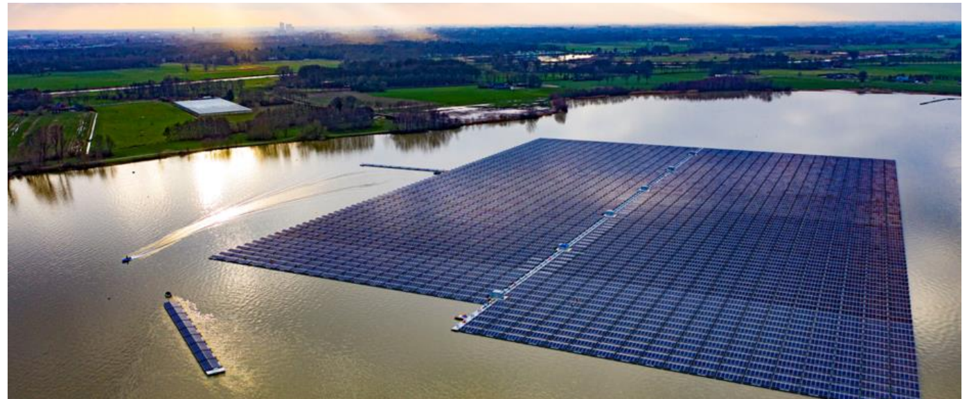
Largest Floating PV system with 27.4 MWp outside of Asia
