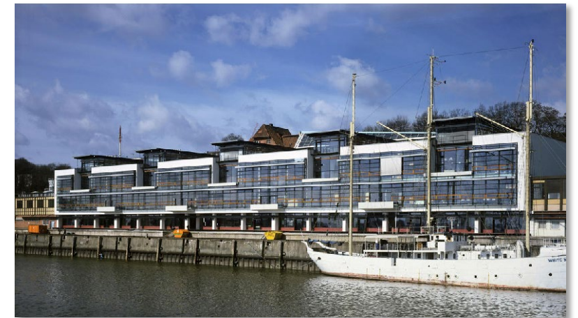
Suntrace Headquarters in Hamburg, Germany
