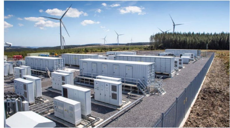
Battery storage at the Pen y Cymoedd Wind Farm in the UK, source: Vattenfall
